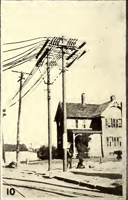
View 5.—Pole shown in views 4 and 5 being raised with pole jacks.
